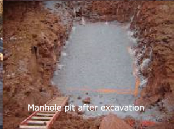
Two manholes next to power lines 13ftx21ftx18ft
