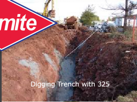
Trench to be drilled alongside the duct bank
