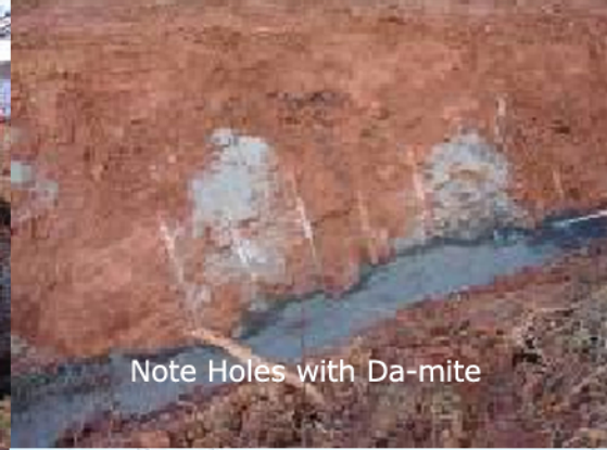
Drilling 2 1/2" holes through 5 feet of overburden
